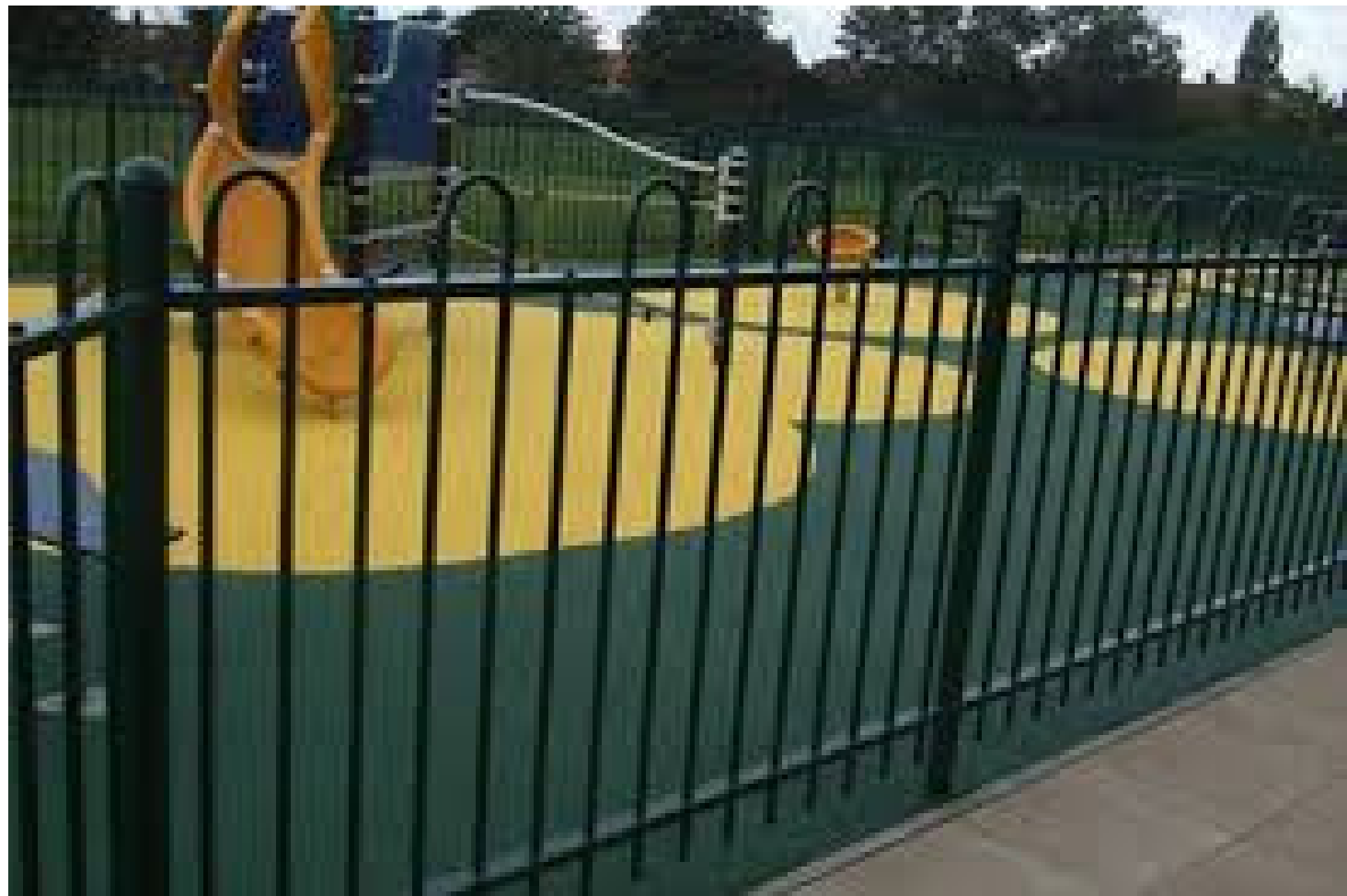
Bow Top Safety Fencing around LEAP
