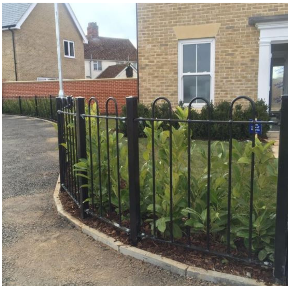
Plot Frontage Bow Top fencing to POS Area
